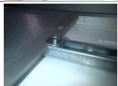
It is better not to fix completely the bar to have the possibility to a final adjustment
