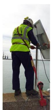
Once the mounting structure is completed, it is possible to fix the solar panel on the top of the pole. In order to facilitate the mounting of the solar panel it is possible to lower the pole to a more easy position and fix the solar panel and bend it at the correct vertical angle, then rise back the pole to its final position, including the right horizontal inclination (normally toward south).
