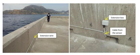
JRC provides the extension cable; this cable is planned to resist to outside conditions. It is however better to consider the installation of a plastic tube that can contain the cable and protect from sun insulation.
