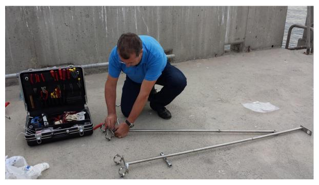
Once the installation of the arm is performed, it can be fixed to the pole using the screws. At this point it is possible to include the sensor and fix the sensor cable using 3 or 4 cable ties (or tie-wraps) along the horizontal pipe.
