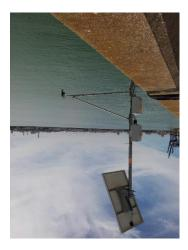
The horizontal angle should be towards south (0). The vertical orientation of the solar panel depends on the latitude of installation. The following table may serve as indication. The orientation can also be computed approximately as follows
