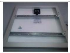
Repeat the same procedure with the other bar and keep a distance between the two bars approximately 50% of the length of the panel. Again do not fix the bars strongly
