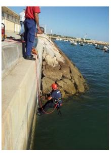
towards the wall by sustaining it with a rope, take the right points where the holes will be made using a marker, remove the pole and finally perform the holes.
