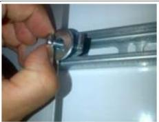
Insert the bolt with the washer positioning the sliding nut inside the bars. Below a detail of the sliding nut. Be careful to position the nut in the direction of closing otherwise it will not fix
