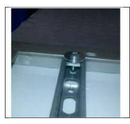
Please note the position of the sliding nuts when blocked in the final position, thy must appear horizontally respect to the bars to avoid to exit
